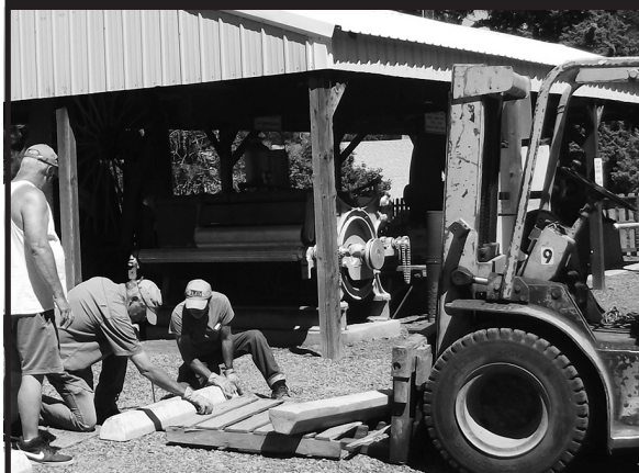
Jerry Warner, Terry Stewart and Ray Cook set the concrete blocks in front of the H&B building.
